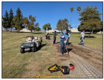
It had been several months since the track gang had replaced a switch; however the skill sets were not lost on the crew. Within two and half hours the new switch was installed ready for the night run later that day.
