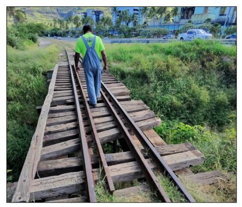
**Left:** The damage done to the bridge track is obvious. Ties out of alignment and it appears maybe a few ties broken that would have to be replaced.
