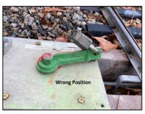
At the last run day I noticed a few locks that were not placed in the "DOWN" position. Severe damage to switchboxes occurs when the lock is standing up. Another reminder to lay the locks down!!!!!!!!!!!!!
