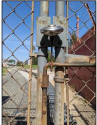
There seems to be some confusion on how to properly lock this gate. When the two gates are pulled closed the "L" shaped handle from the left gate is placed in the "U" shaped tab welded to the right gate. Net you lift the center bar straight up to align all three holes for the lock to pass through. If you are unsure how this works, ask for help. Lately I have been finding it locked improperly.
